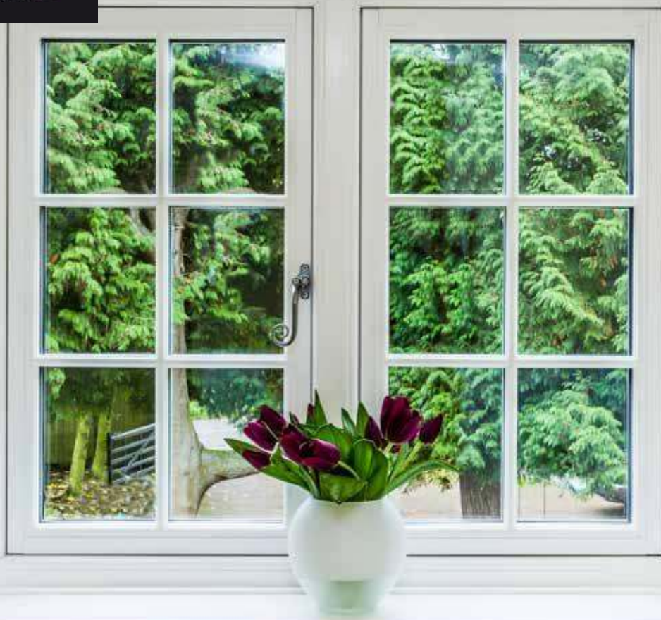
Whitewood Residence 9 windows with feature Georgian bar.
